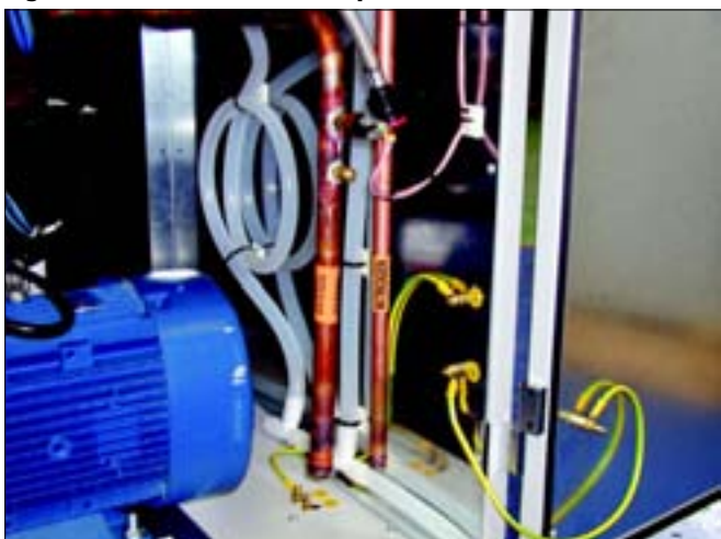
Fig. 1-9 : Condensate drain trap (DX unit shown)
